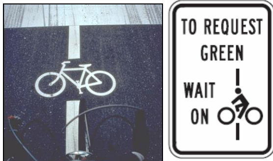
Signal activation marking and sign.
